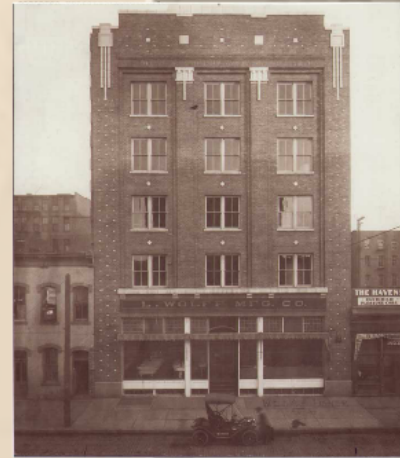
Rockmount Ranch Wear Building
